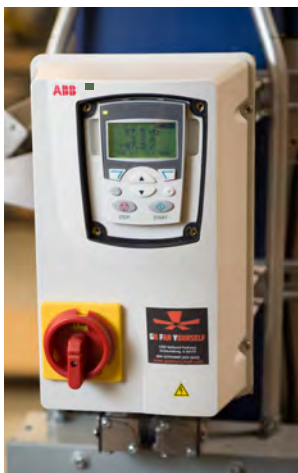
GFY VFD Controller 200-240V & 380-480V 3 Phase
